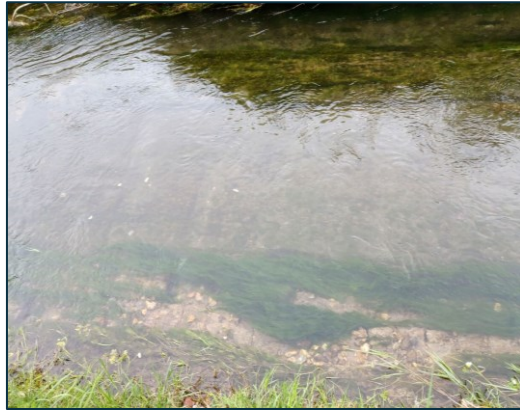
Reinforced bed associated with historical footbridge.
