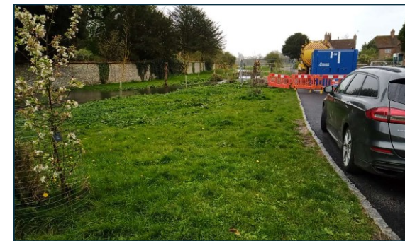
Southern water operatives pumping from network.
