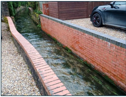
Reinforced banks with opportunity to install gravel bars along banks to create faster flowing mid channel and marginal features
