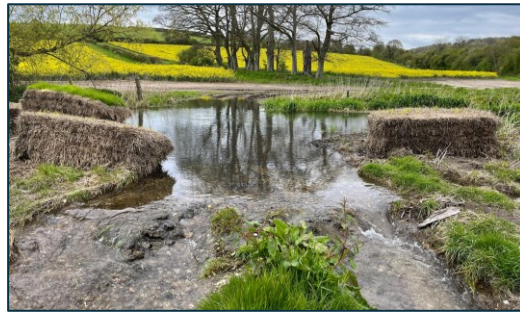
Channel breached at ford.
