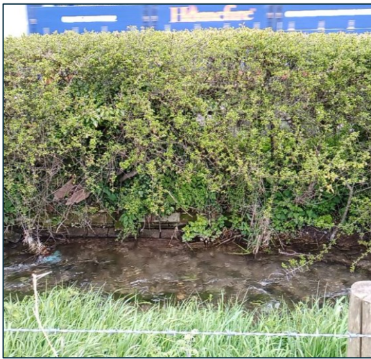
Brick reinforcements along right bank toe.
