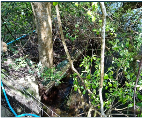
Right bank reinforcement associated with footbridge at start of section (LR14a).
