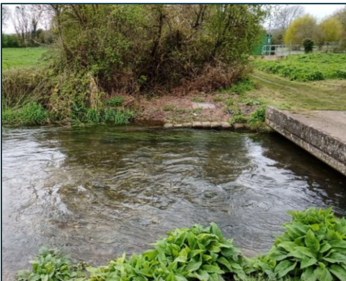
Concrete bridge with reinforcements on right bank
