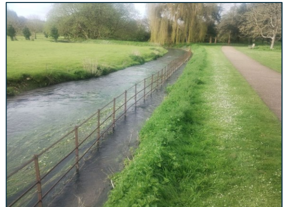
Wet fencing and reprofiled banks upstream of the Pentagon car park.
