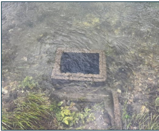
Open drain cover in channel at Farbridge.
