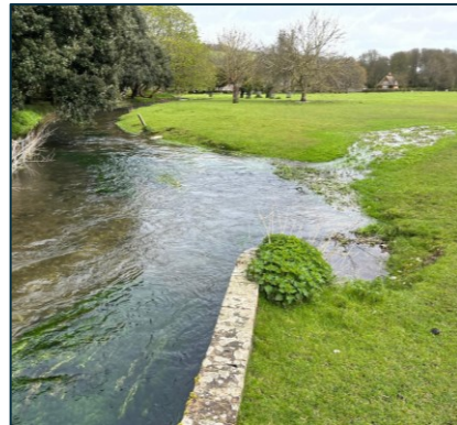
Drain issuing sewage from left bank and reinforced downstream.
