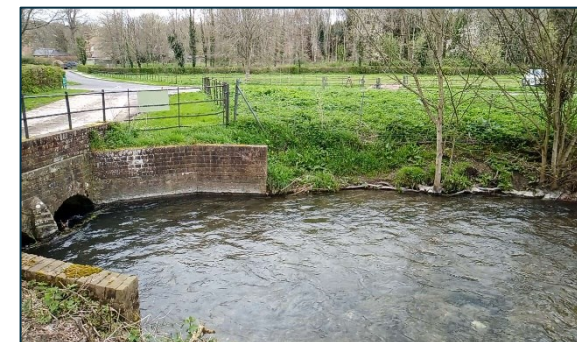
Culvert at downstream end.
